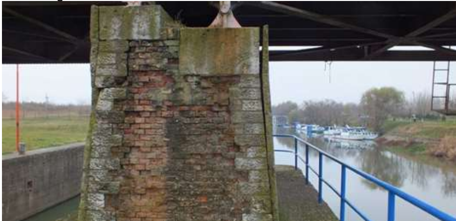
Damaged abutment
