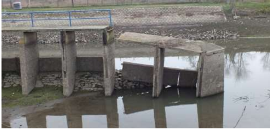
Damaged last two spans of the pier
