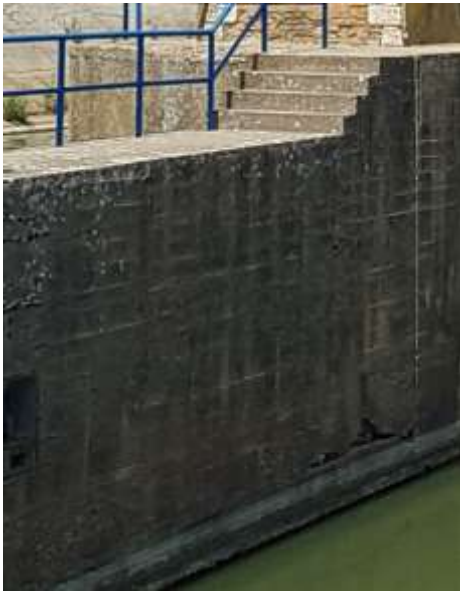
Damaged wall of the lower chamber of the canal lock
