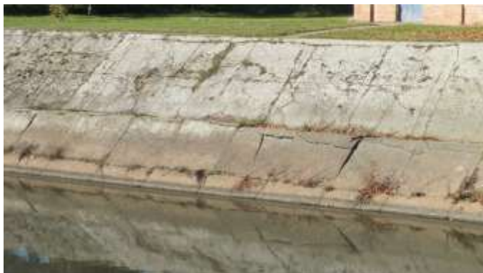
Damaged concrete lining of the canal
